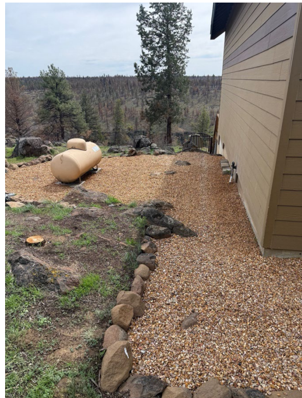
Figure 2. The Flat Fire threatened many homes, including this one, where fire burned close to the structure. Previous mitigation work based on recommendations from the Sisters-Camp Sherman Fire District removed combustibles from around the home and increased defensible space which spared the home from fire damage. Credit: Sisters-Camp Sherman Fire District
